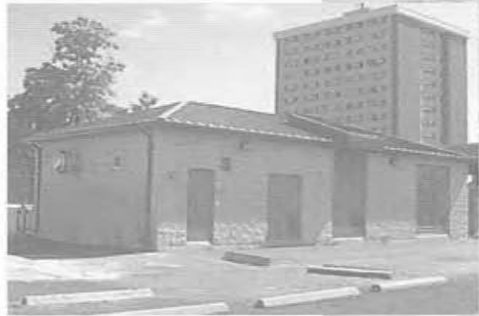
1991: The North Well, a deep well for potable water with a pumping capacity of 1,000 gpm and a 250,000 gallon reservoir, is placed in service on the north side of the MU campus.
