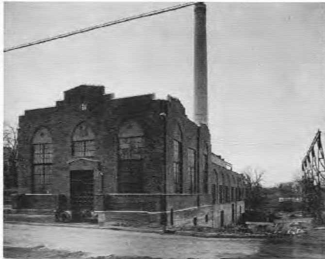
1923: When opened, the power plant had four boilers and two steam turbines. The plant began producing power Jan. 4, 1923.
