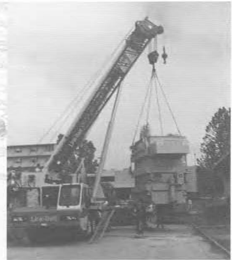
1996: A new, full-capacity (40 MW) 69 kv inter-tie is installed, connecting the power plant's utility lines with the City of Columbia.
