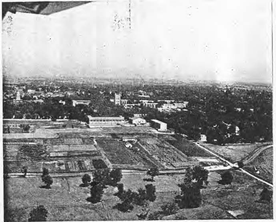
Original site of emergency housing for veterans. In the foreground is shown College of Agriculture experimental fields which gave way to 63 of the 66 Emergency Dormitories for single veterans. Just beyond this site can be seen Brewer Field House, Defoe Hall and Memorial Tower. To the right of the experimental fields, is the site where the faculty housing is being constructed.
